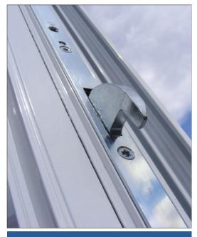
> Hook locking mechanisms as well has shootbolt locking.
